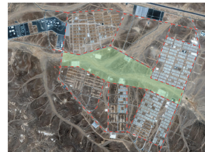
Settlement level (image taken during construction - 11/06/16)
